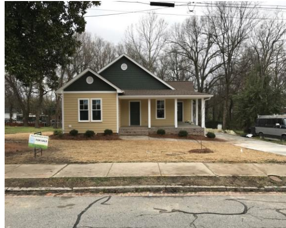
811 Reid Street Ole Asheboro Neighborhood, Greensboro 3 bedroom, 2 bathroom
